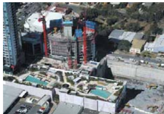
Tower Two emerges (right); the excavated site for Tower Three (left).
